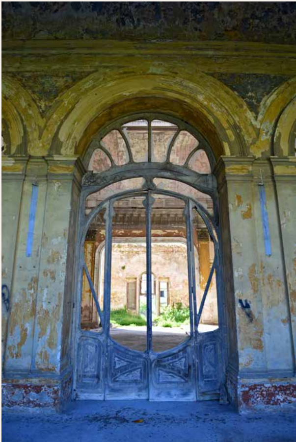
Fig.10 – Porte centrali arcuate in ferro
