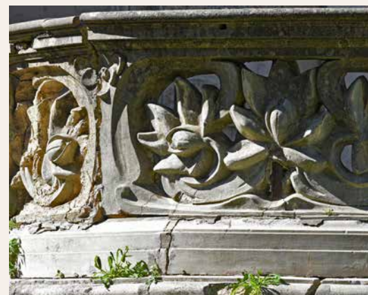
Fig.9 – Balaustra in cemento
